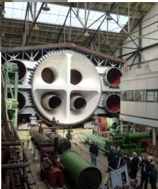
Right: The vacuum/refrigeration plant room and rear of the stratosphere chamber
